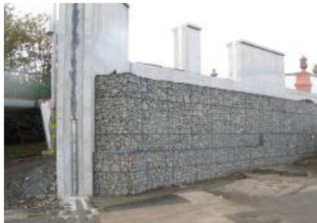
Figure 4.2.3.13: Detail of the finished concrete wall with gabions. Source: T. Drdäcký.
