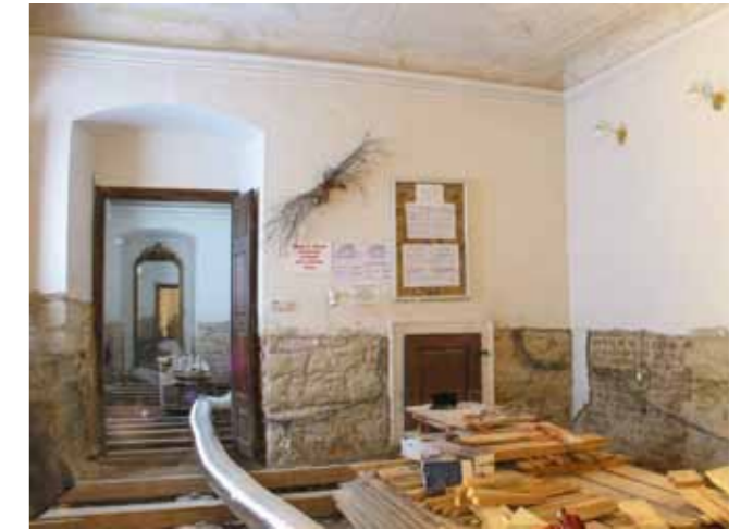
Figure 4.3.3.8: Drying and ventilation of the palace masonry walls. Source: Milan Dropka.
