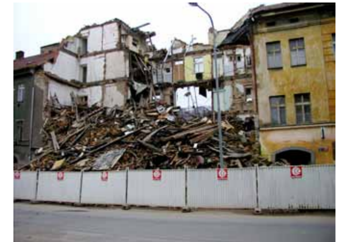
Figure 2.1.2.3: Collapsed building in Karlín. Source: NPÚ, Praha.
