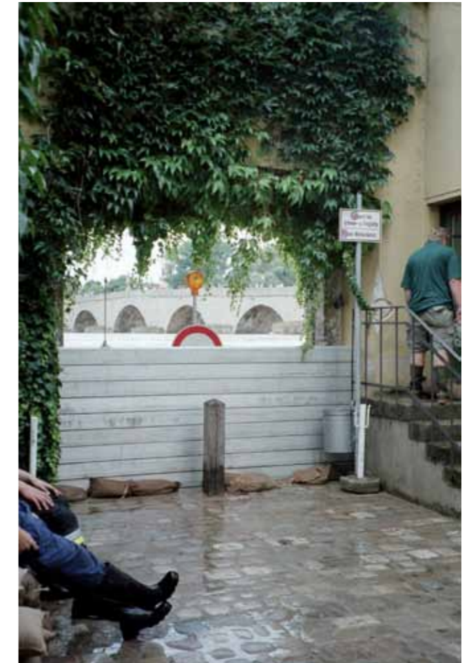
Figure 4.2.2.6 Pictures of the flood in Regensburg in August 2002, with special regard to flood blocking measures. Source: Andy Schwierskott.
