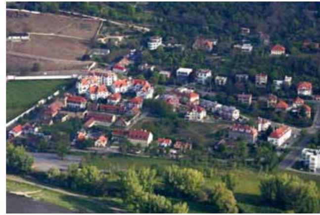
Figure 4.2.3.6: The original situation and the line of the new dike. Source: Municipality of Troja.
