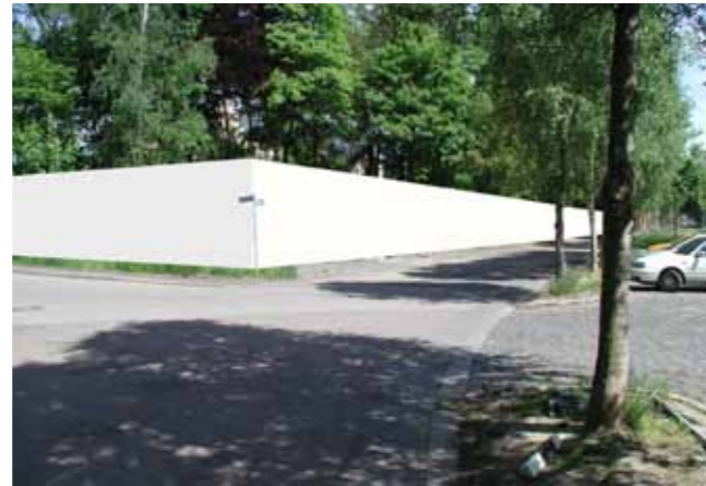
Figure 4.2.5.6: Site of the District Administration Building, monolithic flood protection wall, preliminary planning stage, photomontage. Source: T. Will, H. Lieske.
