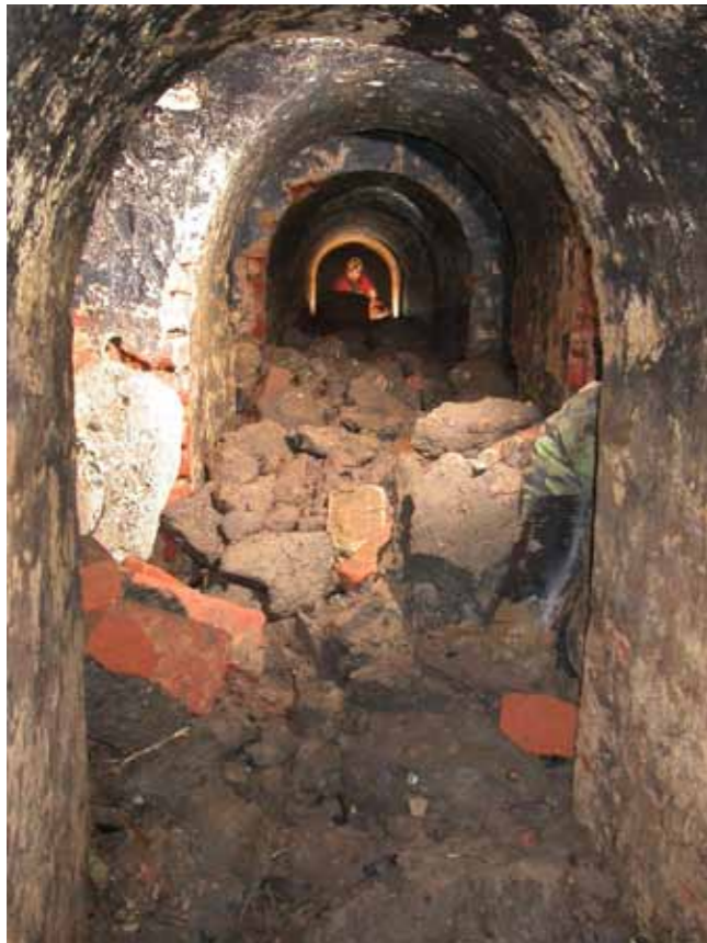
Figure 4.7.1.3: Underground corridors caved with mud and brick (left part), collapsed walls and columns of underground channels. Source: Roman Gazsi.
