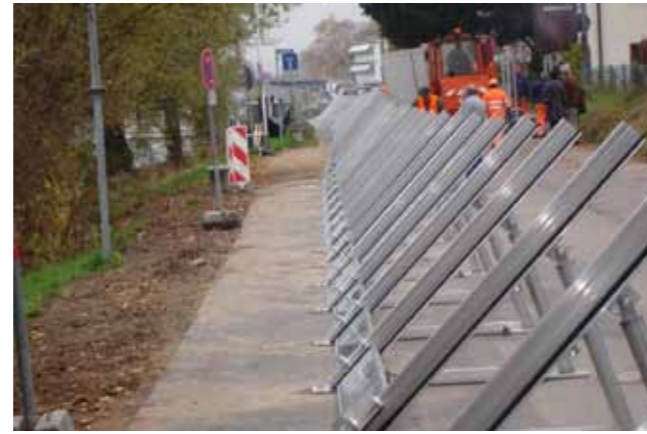
Figure 4.2.2.3: IBS K-system, K-rack fixed with a peg on the pavement (water-side). Source: Xaver Storr.
