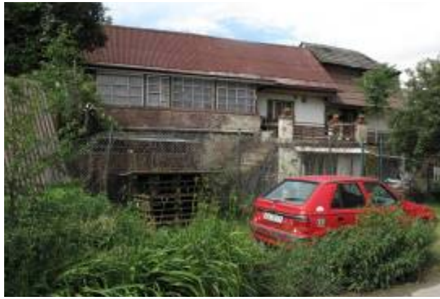
Figure 4.2.3.5: Traditional way of protecting the living area, which is located on the first floor. Source: T. Drdäcký.
