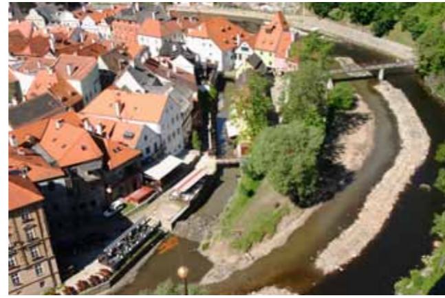
Figure 4.2.6.4: Vltava River during removal work. Source: Klára Nedvědová.
