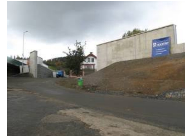
Figure 4.2.3.9: Concrete wall up to 6 m in height. Source: T. Drdäcký.
