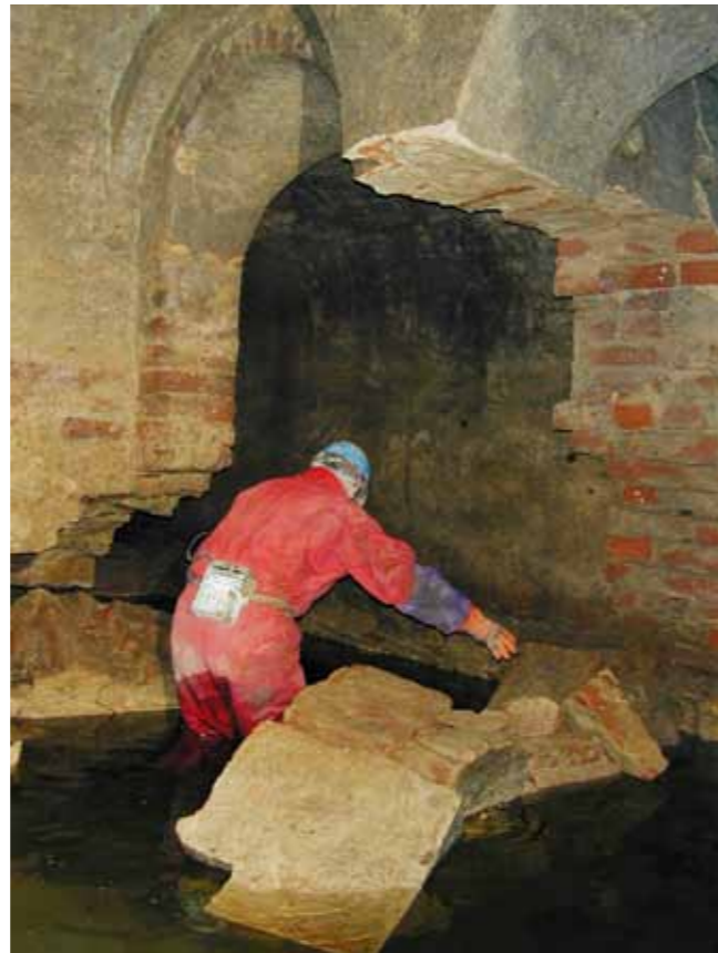
Figure 4.7.1.3: Underground corridors caved with mud and brick (left part), collapsed walls and columns of underground channels. Source: Roman Gazsi.
