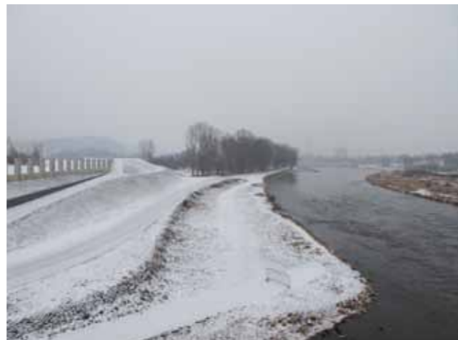
Figure 4.2.3.16: New mound and wall separating the area next to the river from the inner part of the district. Source: T. Drdäcký.
