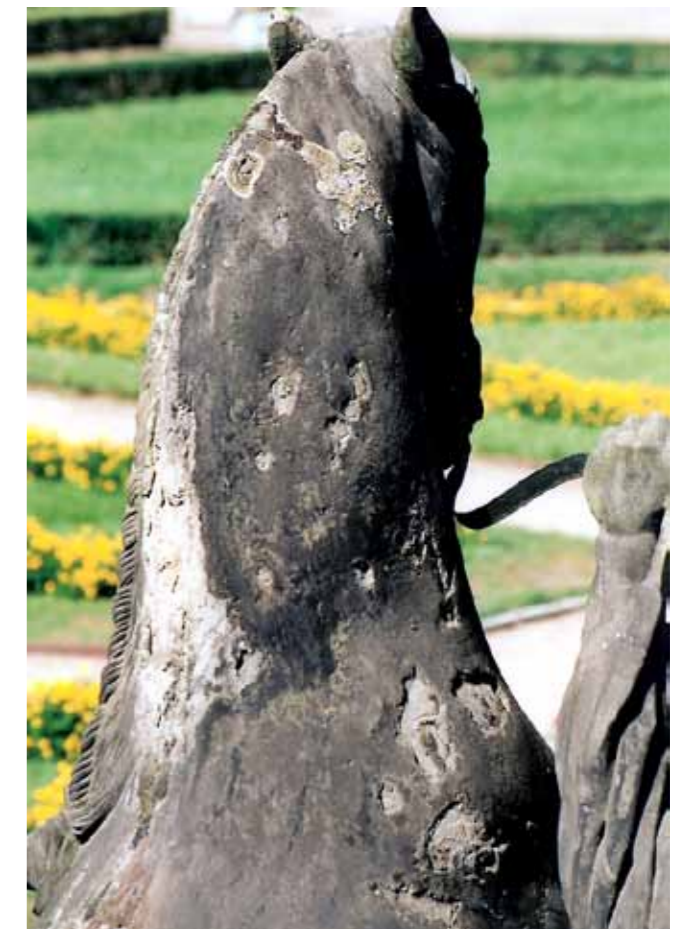
Figure 4.3.3.5: Incorrectly restored sandstone sculptures. Source: Vojtěch Adamec.
