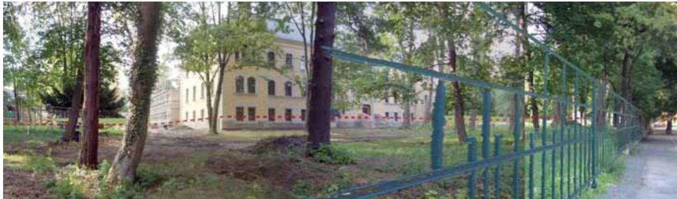
Figure 4.2.5.7: Site of the District Administration Building, dotted line indicating flood protection integrated into the historic building. Integrated planning proposal, photomontage. Source: T. Will, H. Lieske.
