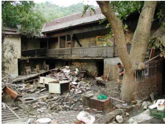
Figure 4.1.1.3: The high-water level is visible on the roof. Source: M. Drdäcký
