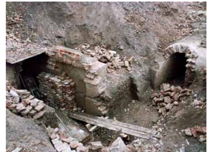
Figure 4.7.1.5: Repairs to shallow mine corridors (left), and to damaged vaults (right). Source: Roman Gazsi
