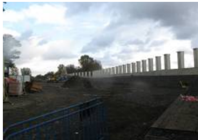
Figure 4.2.3.14: Concrete wall from the village side. Source: T. Drdäcký.
