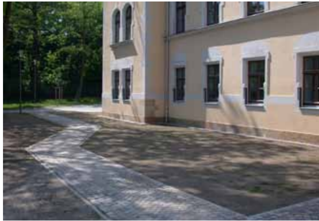
Figure 4.2.5.5: District Administration Building, flood protection integrated into the historic building, 2009 (note the U-profiles in the window reveals, with covers temporarily removed, to hold stop logs). Source: T. Will, H. Lieske.
