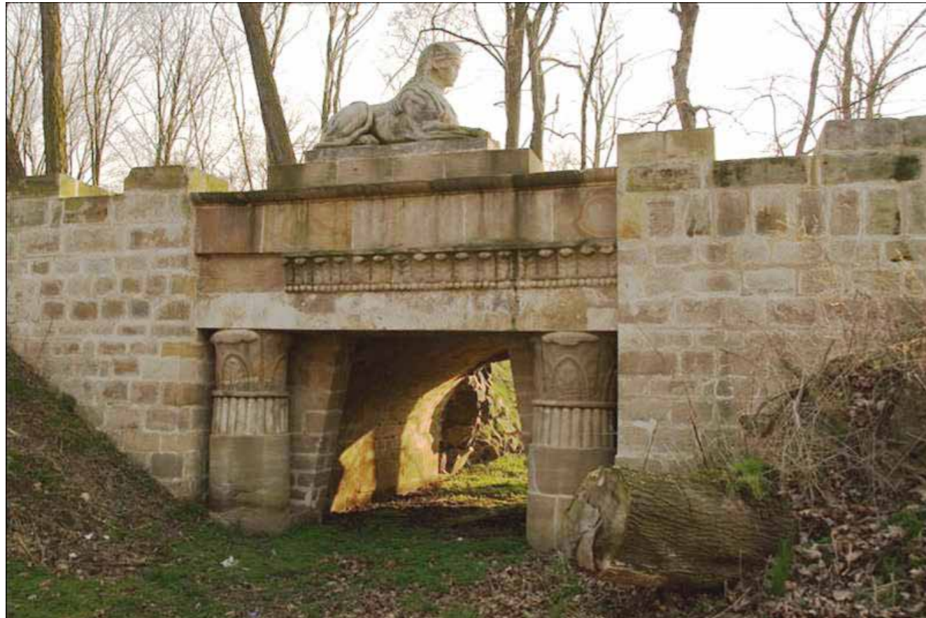
Figure 4.3.3.6: Restored bridge before the flood. Source: Vojtěch Adamec.
