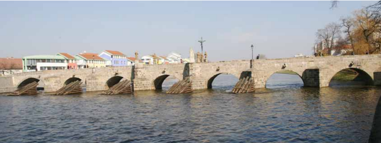
Figure 4.4.1.1: Stone bridge in Písek after restoration following the disastrous flood in 2002. Source: M. Drdäcký.
