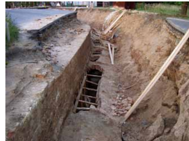
Figure 4.7.1.5: Repairs to shallow mine corridors (left), and to damaged vaults (right). Source: Roman Gazsi
