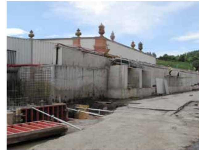
Figure 4.2.3.7: Difference between the scale and detail of the historic wall of Troja Chateau with decorative terracottas and the new concrete wall. Source: T. Drdäcký.
